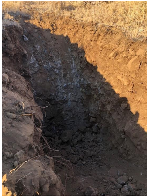
Completed test pit.
