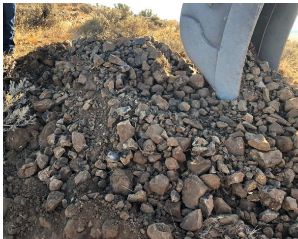
Test pit spoils.
