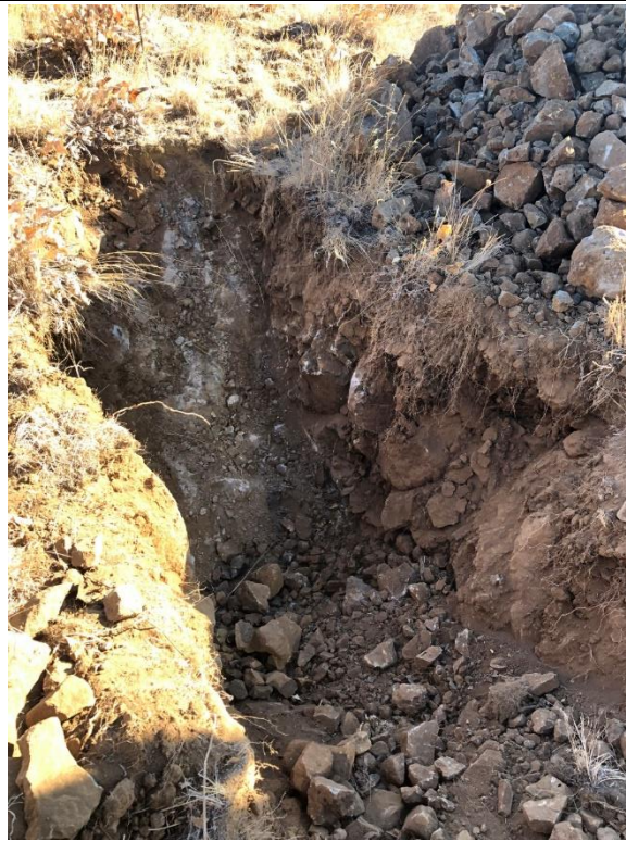
Completed test pit.
