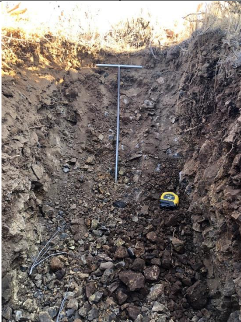
Completed test pit.
